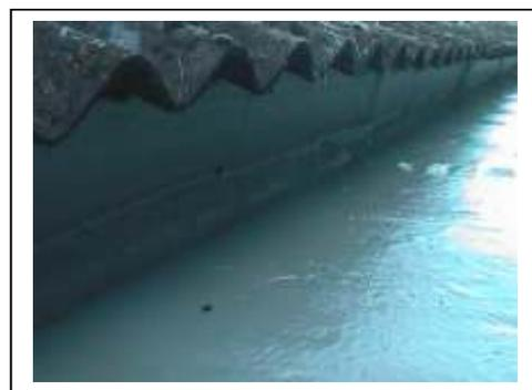
Above a typical tin/zinc lined valley, used over many years in agriculture, commercial and industrial buildings. Over the years the metal surface has badly rusted and delaminated, causing weakness to its structure and then allowing water to penetrate the structure within causing untold damage to the contents within the building.
