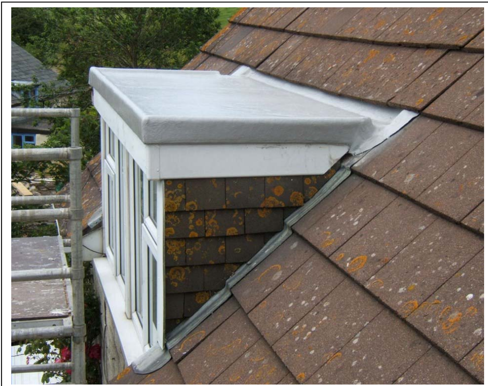
Above, The original felt covering has deteriorated and leaking badly.
