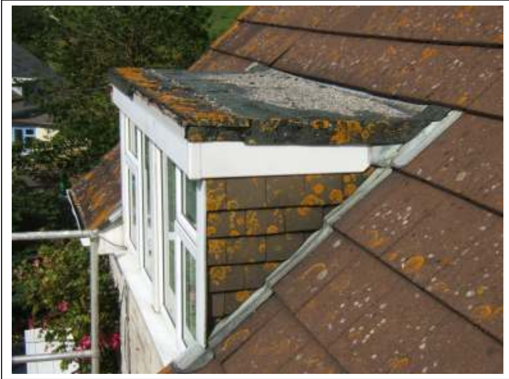
Above, The original felt covering has deteriorated and leaking badly.
