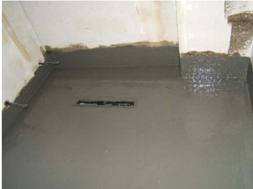
Above: GRP Wet Room System installed.
